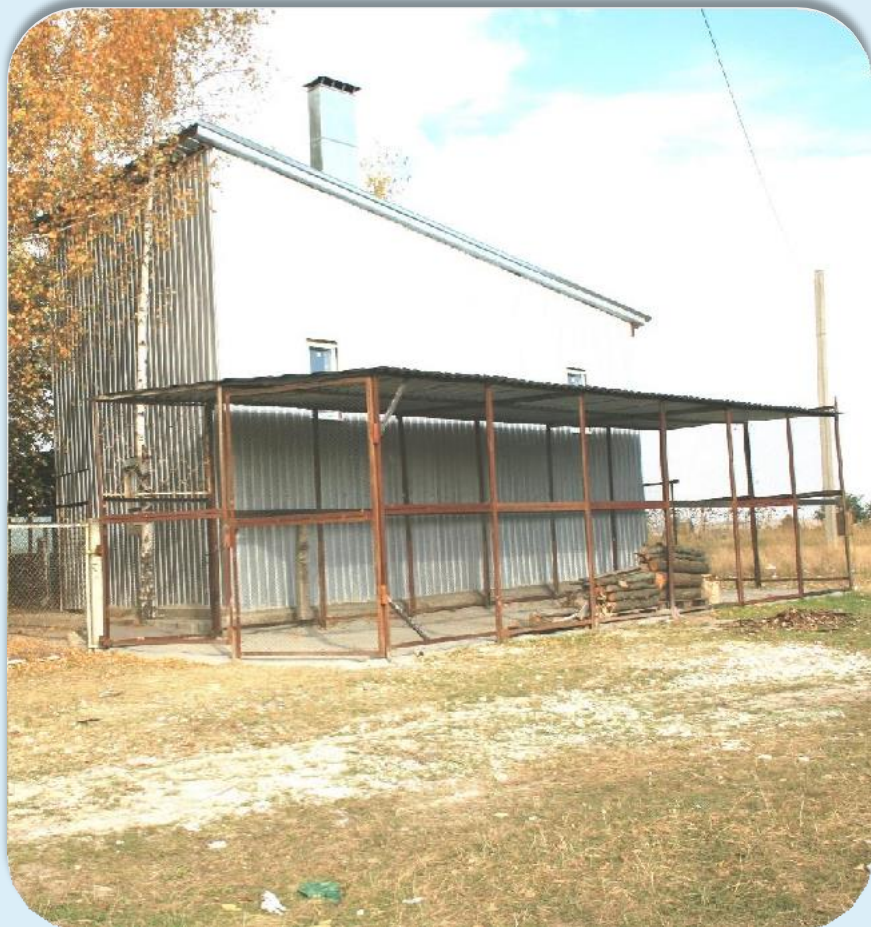
Heating Device 1,2 MW
