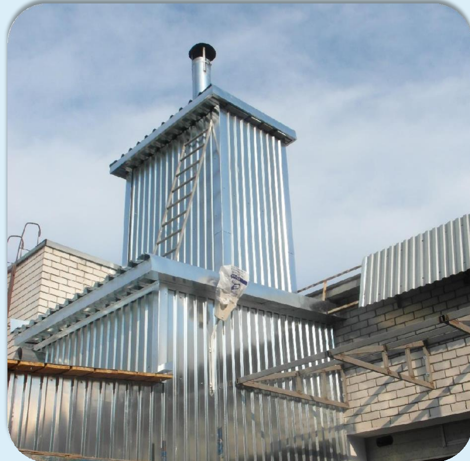
Heating Device 1 MW
